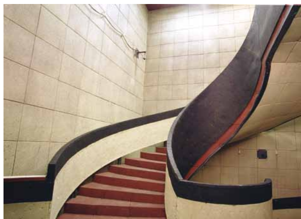
The GSG 9 shooting range in Hanglar (Germany) is completely covered with Regupol® Elastic Tiles E43 .
